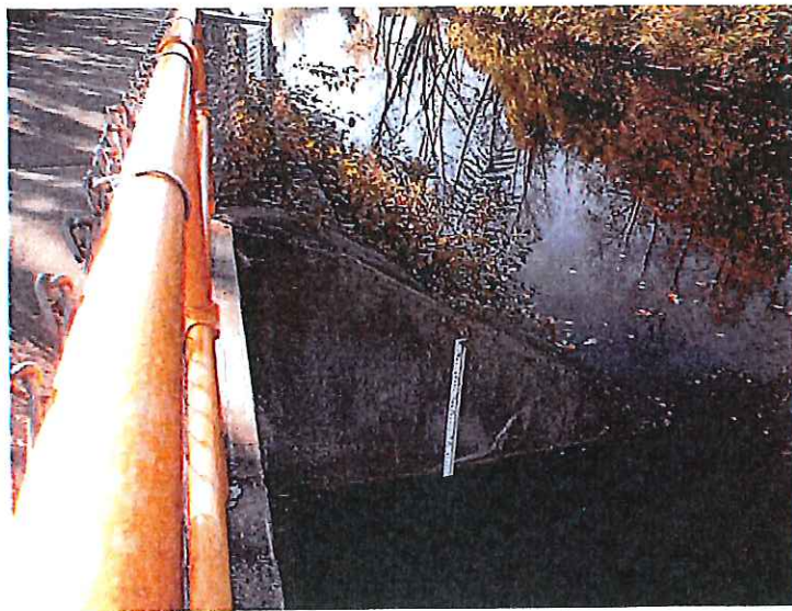
11. Staff gauge found on the right sidewall of the spillway inlet.
