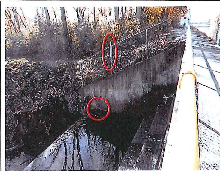
10. Right sidewall of the spillway.
