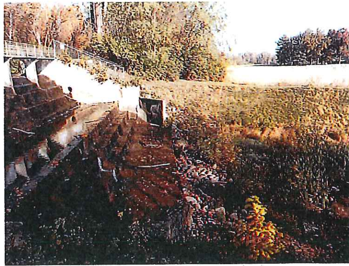
9. Left sidewall of the spillway.
