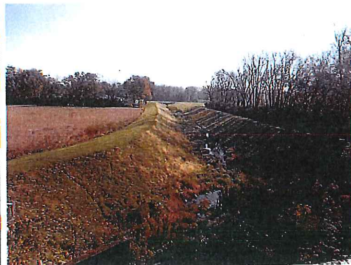
12. Outlet channel for the spillway.
