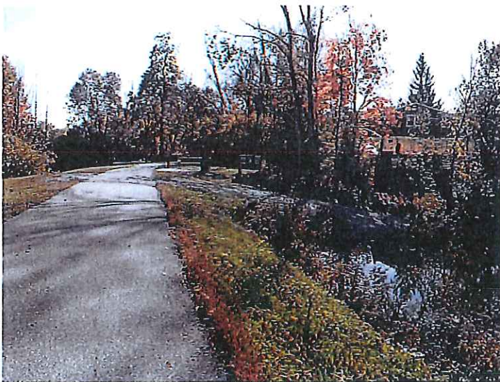
3. Right end of the dam.
