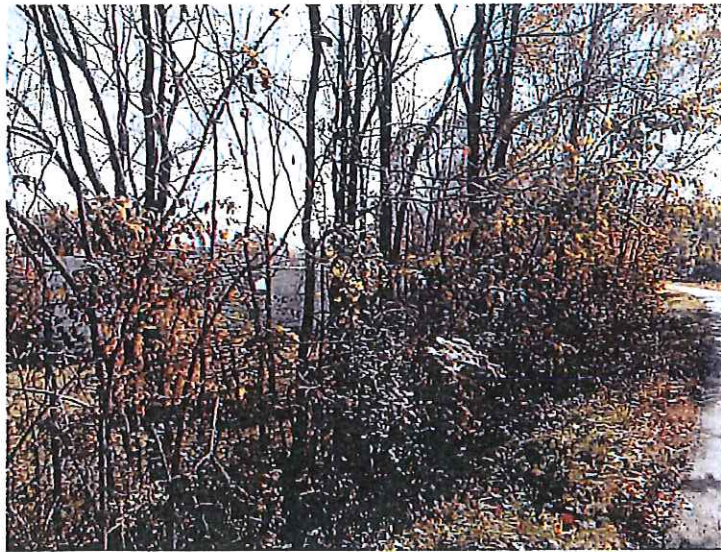
5. Downstream slope. Note the dense trees and brush.
