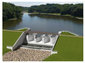
The footprint of the proposed spillway would vary depending on the normal pool elevation within Swift Run lake post construction. Should the normal pool elevation remain the same, the labyrinth will likely fill the entire length of the embankment from Spillway 2 to Spillway 3. If the City can drop the normal pool elevation at Swift Run lake the proposed footprint will decrease.
