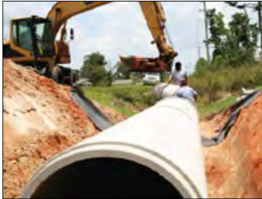
Storm Sewer Re-Routing / Diversion
