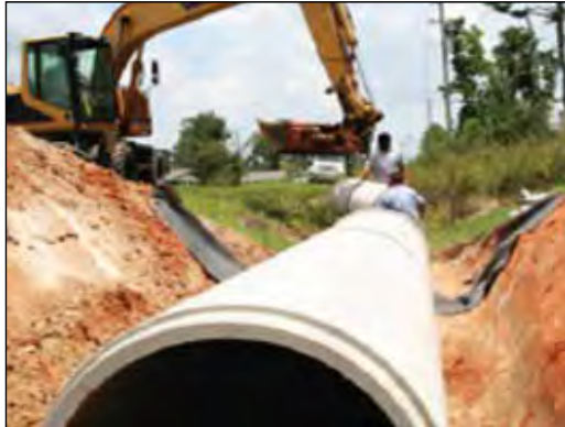
Storm Sewer Re-Routing / Diversion
