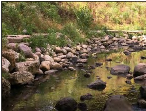
In-Stream Bank Stabilization
