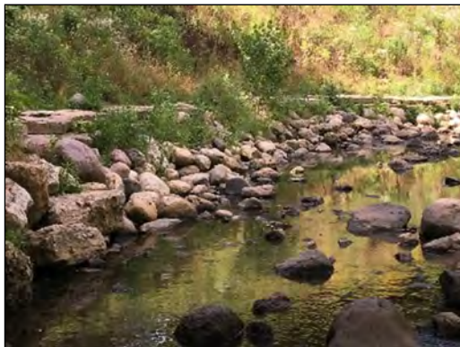
In-Stream Bank Stabilization
